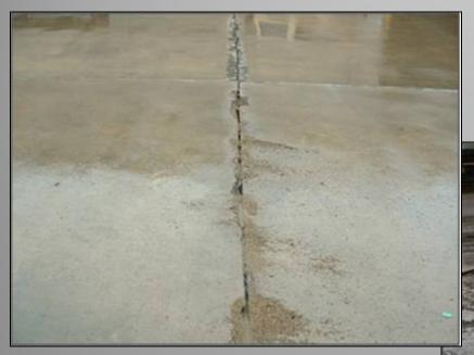
Pumping of fines causing voids to form
