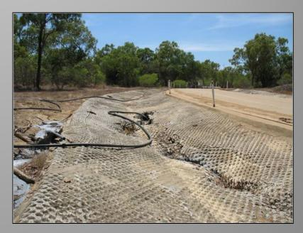
This grouting saved catastrophic failure during the wet season
