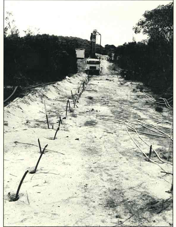
Installing the grout wall
