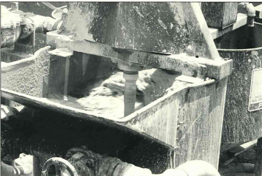
Mixing the grout
