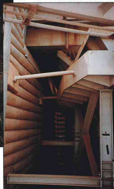
The narrow void in which the work was carried out.
